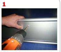
drill through the rivet until you're able to remove the pole bucket
